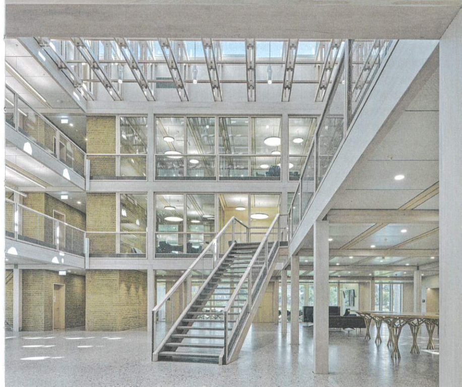
A timber structure, robotically manufactured rammed earth cores and a prototype hybrid floor/ceiling system define Erne's timber branch extension of 1500 m 2 of floor area in doubling the size of their team: Erne offices extension (Stein, Switzerland, 2023).
